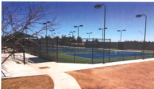
Westwood Tennis Center Improvements
