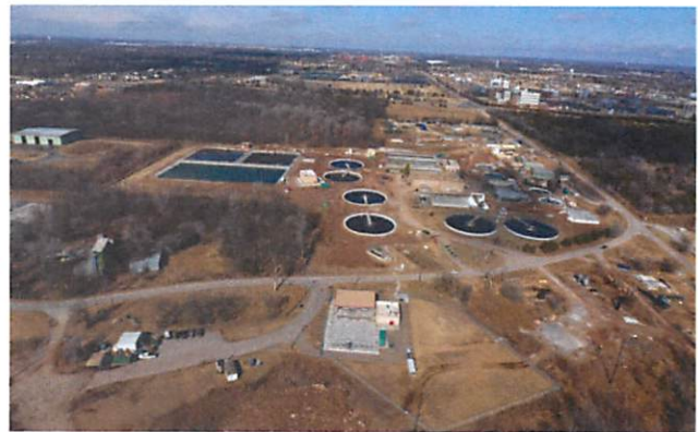
Water Reclamation Facility Expansion
