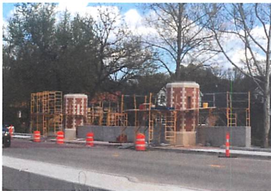
Lindsey Street Bridge over Imhoff Creek
